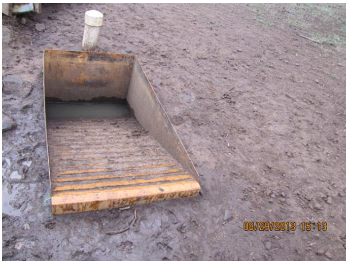
Storage tank is possibly cracked
