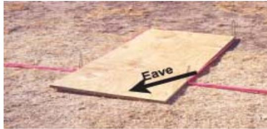
Backer board moved 10" forward to create the eave, with rope creating an outline around the 3 sides of the backer board
