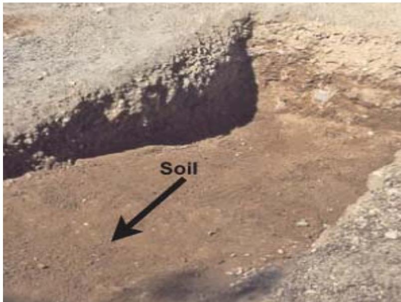
The ramp (where the roof will rest), before the channel has been dug
