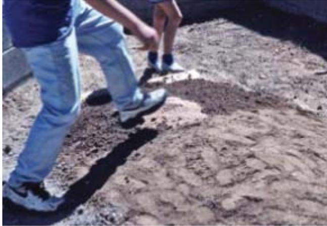
Creating the mound of insulating soil on the top, sides, and back of the burrow
